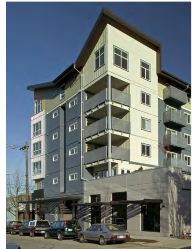
Communal Balconies, Denny Park (above)
