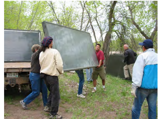
Reclamation of a Previously Owned Solar Hot Water System, Wild Sage
