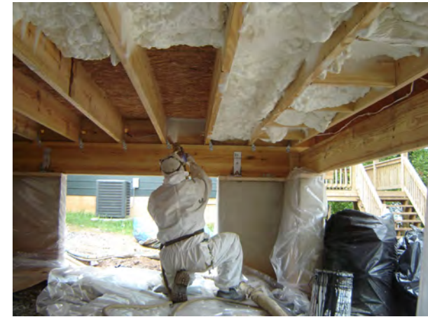
Icynene spray foam insulation installation, ecoMOD3
