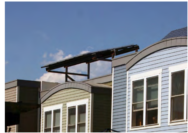
Owner installed PV rack , Wild Sage
