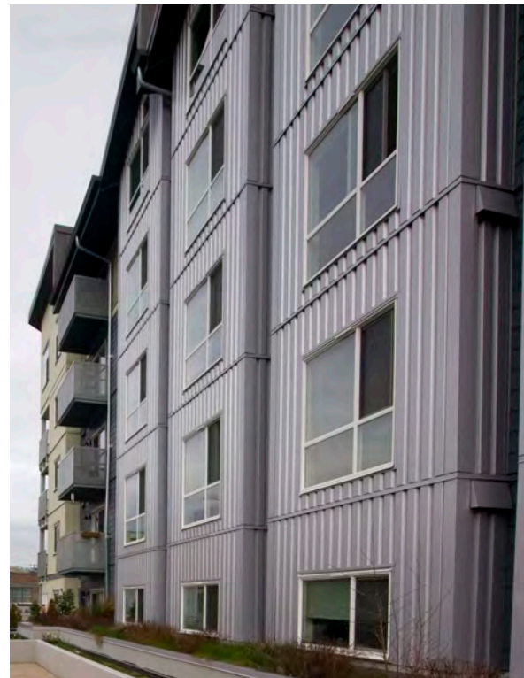
Low-maintenance metal cladding, Denny Park
