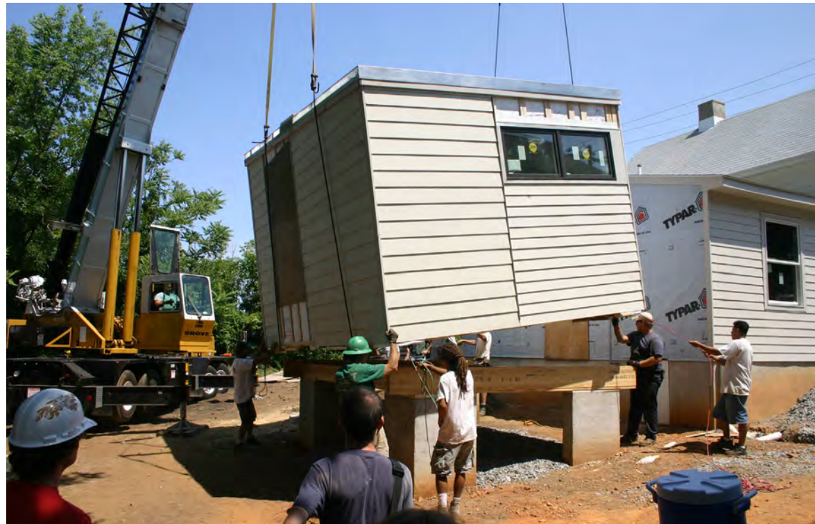
Module Placement, ecoMOD3
