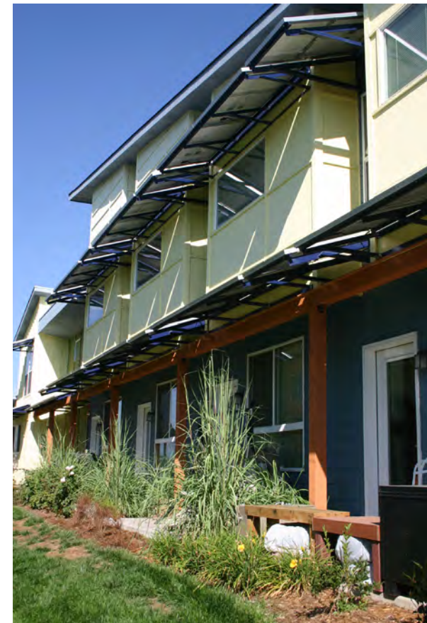
Building Integrated PV sunshade, Eagle Place
